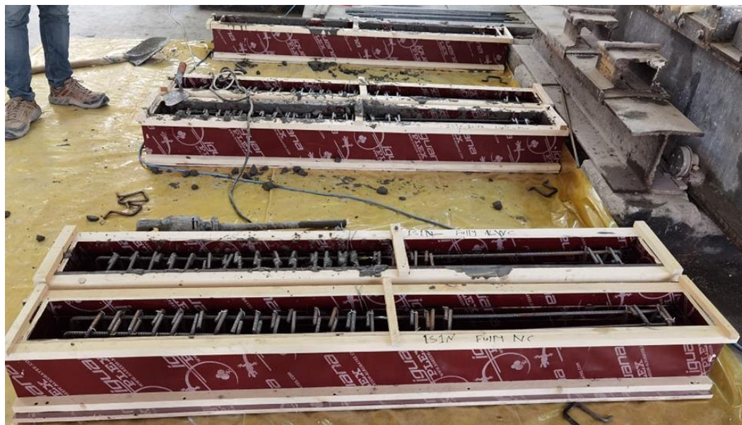
Fig. 4 Plywood forms, steel placing and concrete casting.
